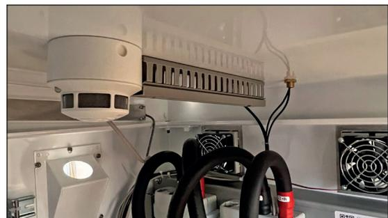
Fig. 37: Position of smoke switch
