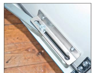
Fig. 13: Unlocked door latch
