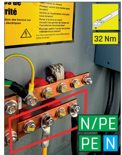
Fig. 33: Connection main AC supply N/PE
