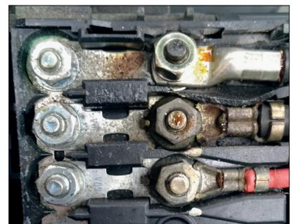
Fig. 34: Example of a defective connection terminal, visible by discoloration.
