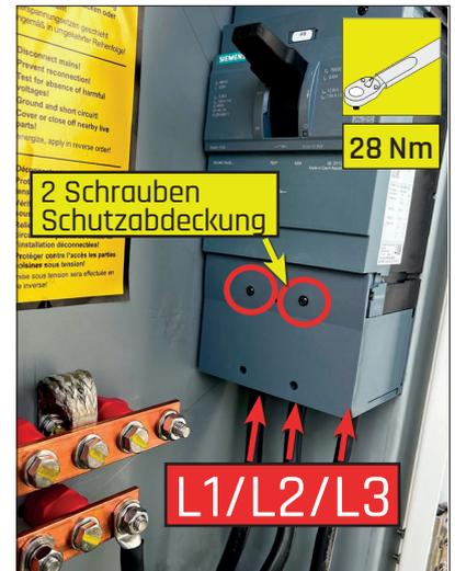
Fig. 35: Connection main AC supply L1/L2/L3
