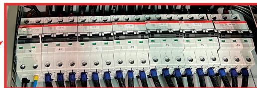
Fig. 23: Line/fault-current circuit breakers
