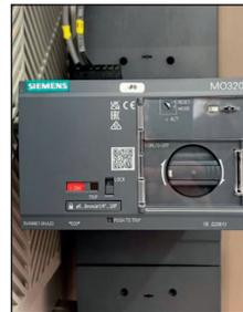
Fig. 55: Motorized switch disconnecter
