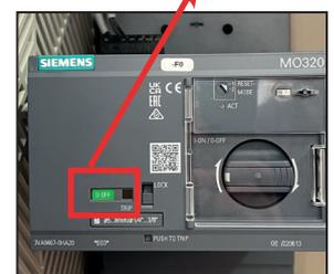
Fig. 26: Motorized fuse-switch disconnecter
